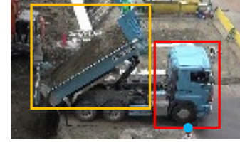
[Legend] □ : movable part, □ : vehicle body, ● : position coordinates of construction machinery
